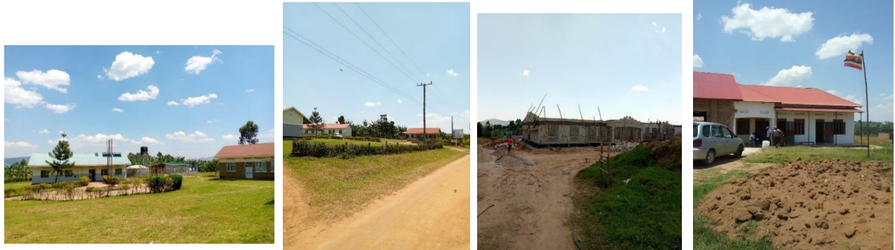
From Left: maternity ward, staff housing and outpatient units, the new health center under construction (by Sheema District Local Government) and the new Kyeibanga Subcounty headquarters.
