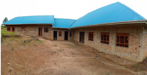
The HC under Construction
